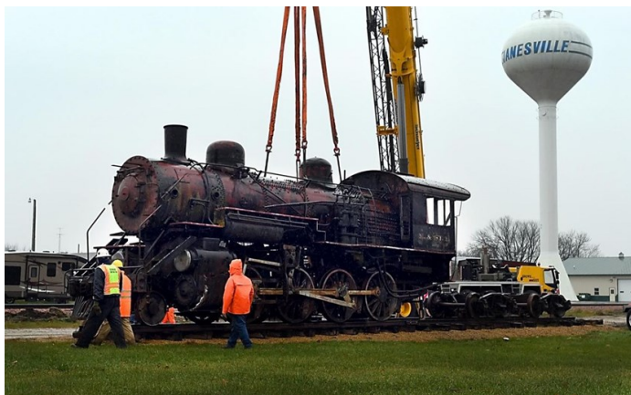
A crane lowers a locomotive boiler onto its wheels Tuesday in Janesville. Photo by Pat Christman
